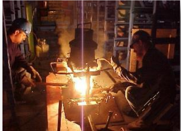
Thermite Welding AS/RS Rail Repair Procedure
