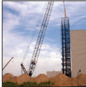
Begin Rack Erection
