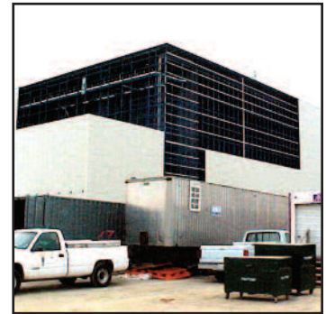
Complete Siding and Roofing
